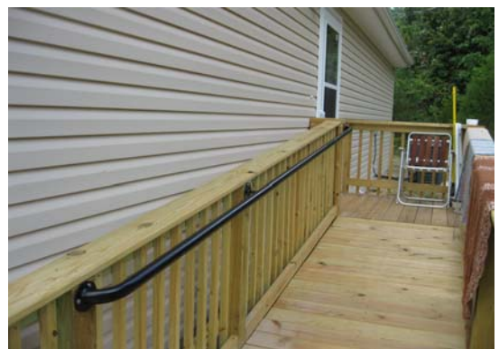
Handrail along ramp
